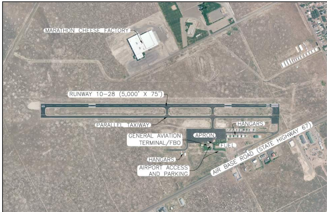
FIGURE 2-2 – AERIAL OF AIRPORT FACILITIES
