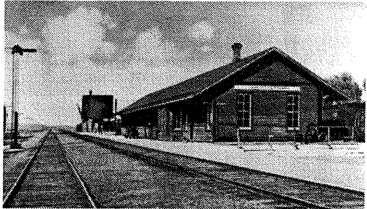
Former Mountain Home passenger depot and water tank. (ISHS P1987.0006.0001)
