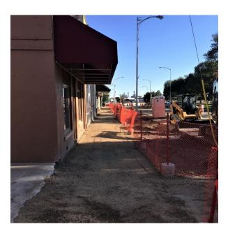
Sidewalks along Main Street have begun the demolition phase, beginning with the first block between East Jackson Street and East 2nd North Street. The first block now has a temporary, ADA compliant, compacted gravel sidewalk 6 feet out from the building face. Crews have also finished the demo of the sidewalks to the curb and have separated the sections by an orange safety fence to delineate pedestrian walkways with work areas.
