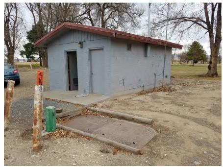
The building is old and had many changes and modifications over the years. Due to the removable roof and wall section for well access, the building is subject to increased deterioration from weather and water intrusion.
