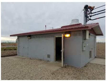
site is fenced with a gate at the road. Power is overhead from a power pole near the road. SCADA system and an antenna on pole next to the roof provide remote monitoring.
