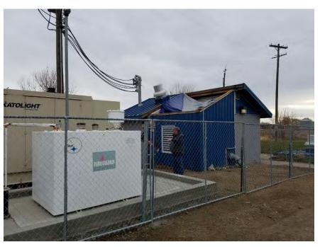
generator is located in a fenced area nearby. An additional secondary containment curb has been added to the aboveground fuel tank since the double wall fuel tank was installed years ago. The pump and motor assembly was under repair at the time of the evaluation. The motor was scheduled to be reinstalled soon. The roof section over the pump was removed and covered with a tarp. The roof is removal for pump maintenance. The roof will be replaced after the pump repair is complete.
