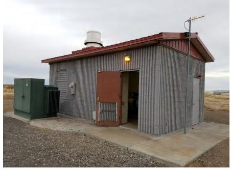
control system. The pump is cooled with a roof fan and louvers. The louvers are boarded up during the winter. No standby power at this well. The site is fenced. The pump waste discharge flow out onto the ground.
